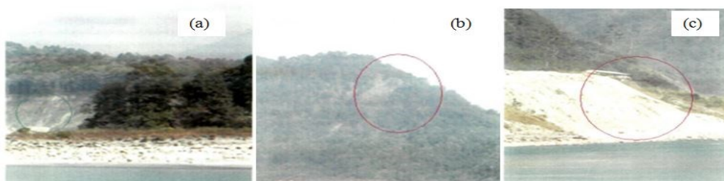
Fig. 2. Landslide (a) Due to Excessive Rainfall at Rambi Bazar (b) Due to Removal of Vegetal Cover at Labda Khasmahal and (c) Beside the Bank of Rayeng Near Confluence
